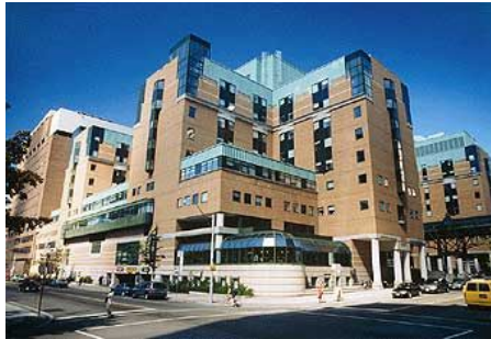
The Hospital for Sick Children – Atrium Wing Toronto, Ontario, Canada
